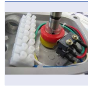
technical switch N.O. / N.C. SPDT make Honywell, type ZM50D
